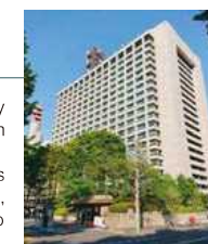
Central Gov't Bldg. No.2
